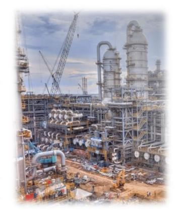
Usually, between 60 and 70 percent of the scope is self-performed work by SHATHCO specialists. Such works include Civil works, Steel structures, Concrete works, Plate and duct works, Demolition, Installation of piping and process equipment, etc. The company approach has proven the greater control of safety, quality, schedule, and cost of the project.
